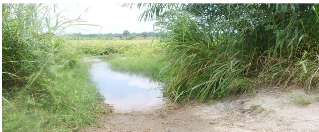
Photo 10: Main community dam at Xevi, almost fully covered with plants
