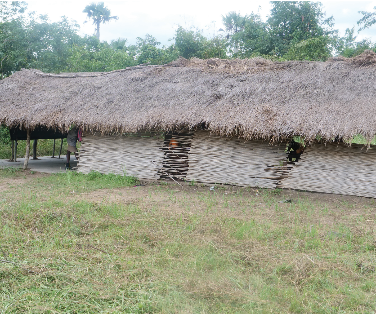
Plate 7: The only community primary school Credit: Portia Adade Williams and team, 2024
