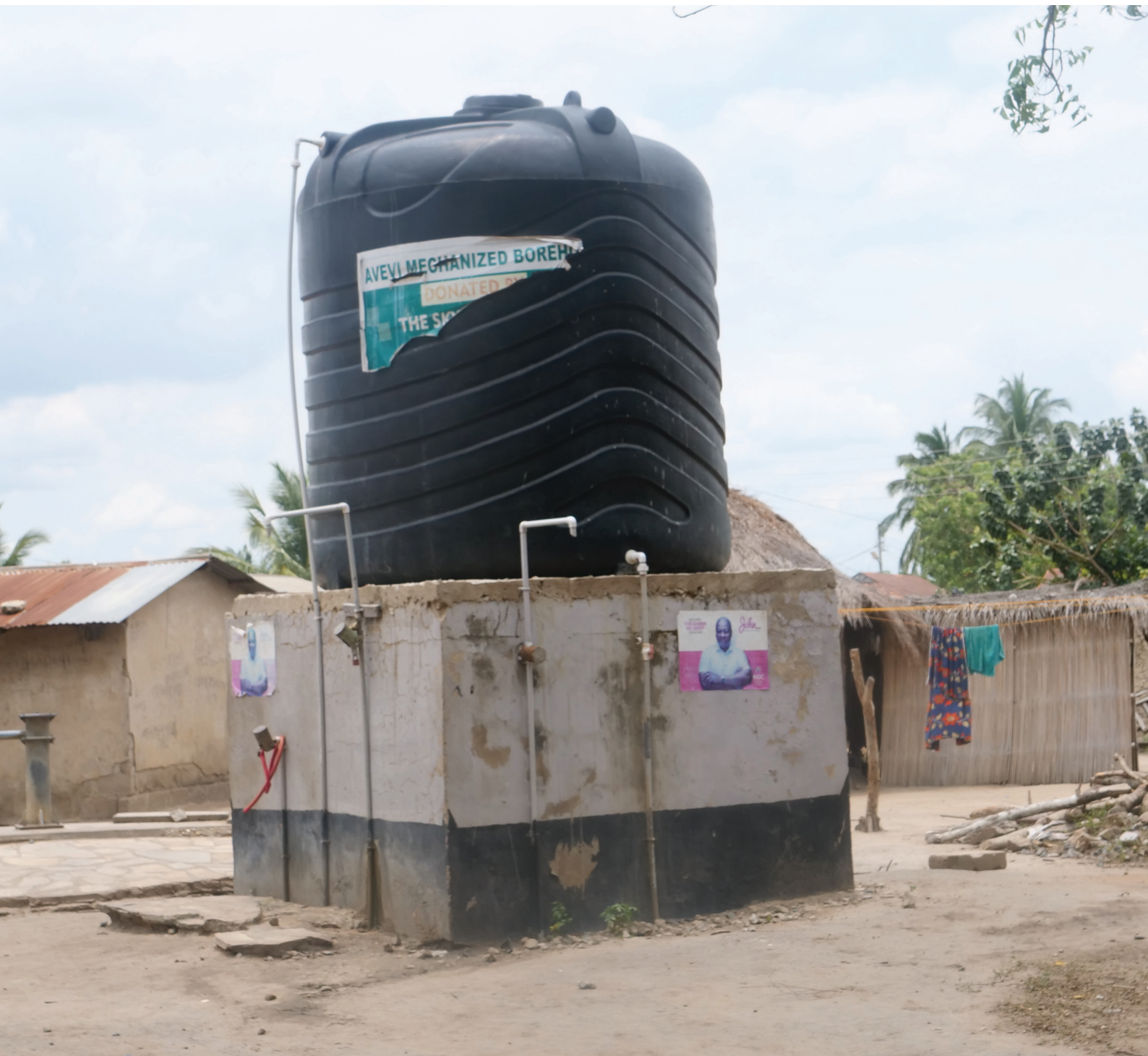
Plate 8: Avevi only community mechanized borehole Credit: Portia Adade Williams and team, 2024
