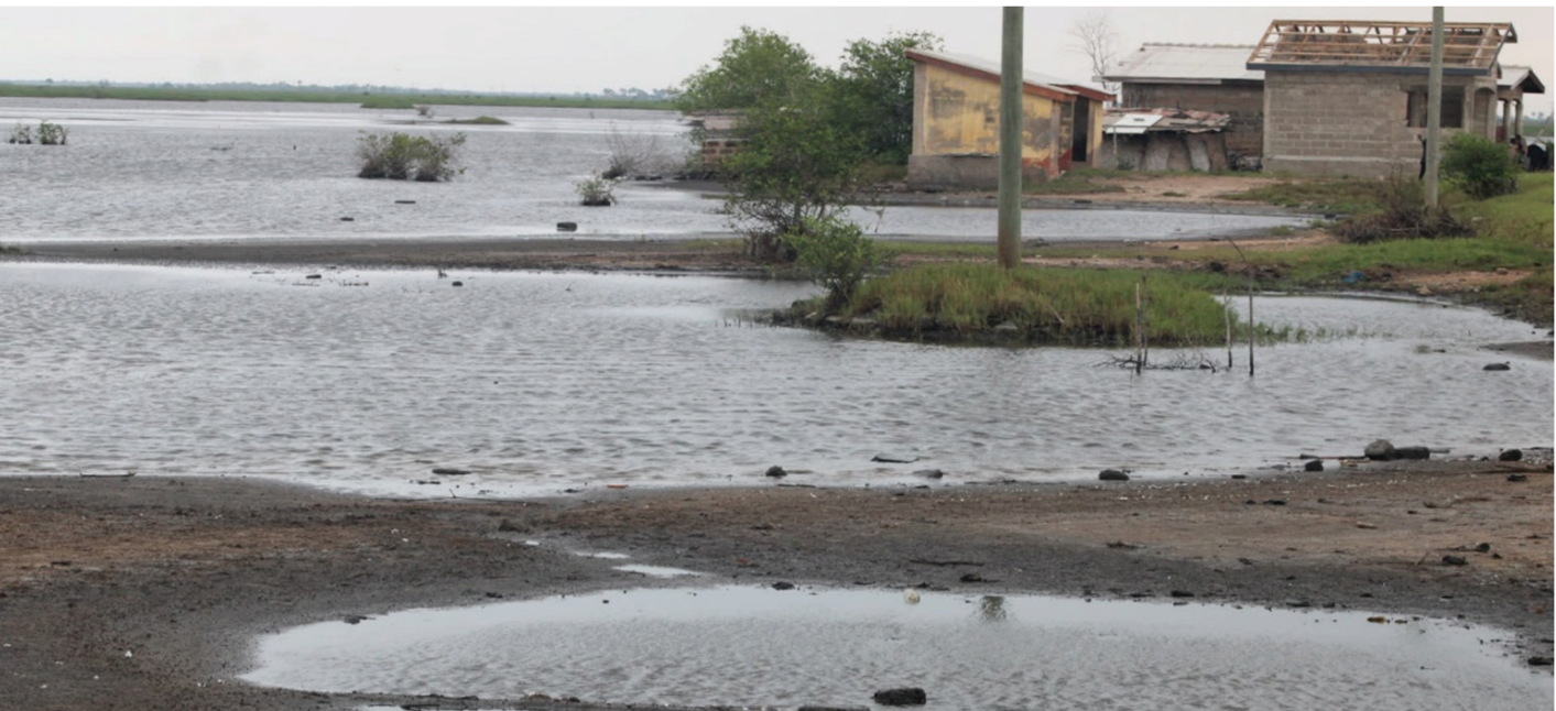
Plate 2: Flooding situation at Atito-Alakple Credit: Desmond Adjaisson, 2024
