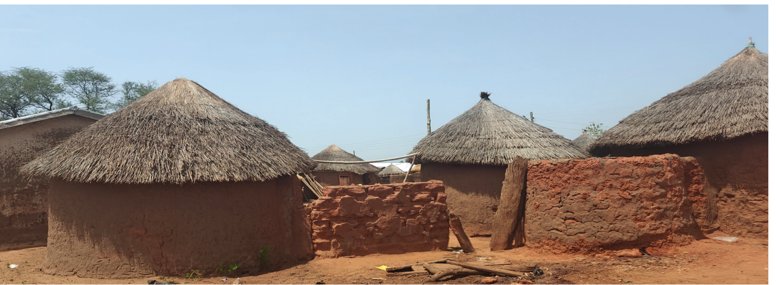
Plate 2: A view of a typical home in Mion, featuring traditional mud-and-thatch roundhouse. Credit: Cephas Adorliyah, 2024
